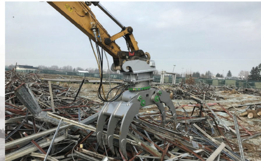
Demolition of steel structures and safe gripping of sharp steel profiles with the "Alligator" shape.
